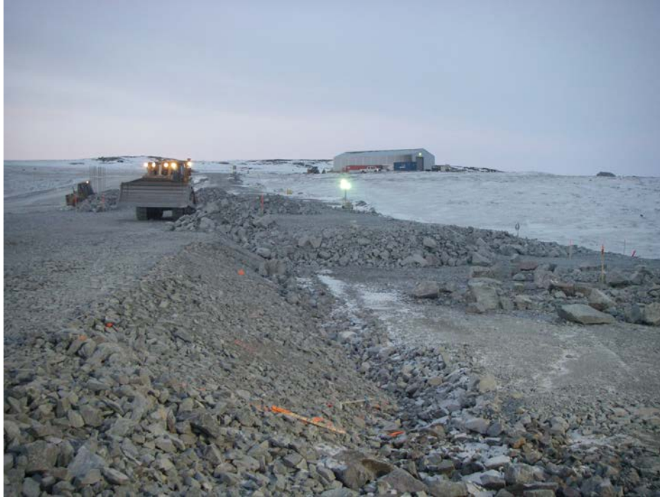
Photo 10: North Dam – CAT D8 dozer placing the third lift of ROQ. Note the boulders spread out in the right side of the photo, to prevent creation of large cavities. Photo looking north-east from Sta. 0+40
