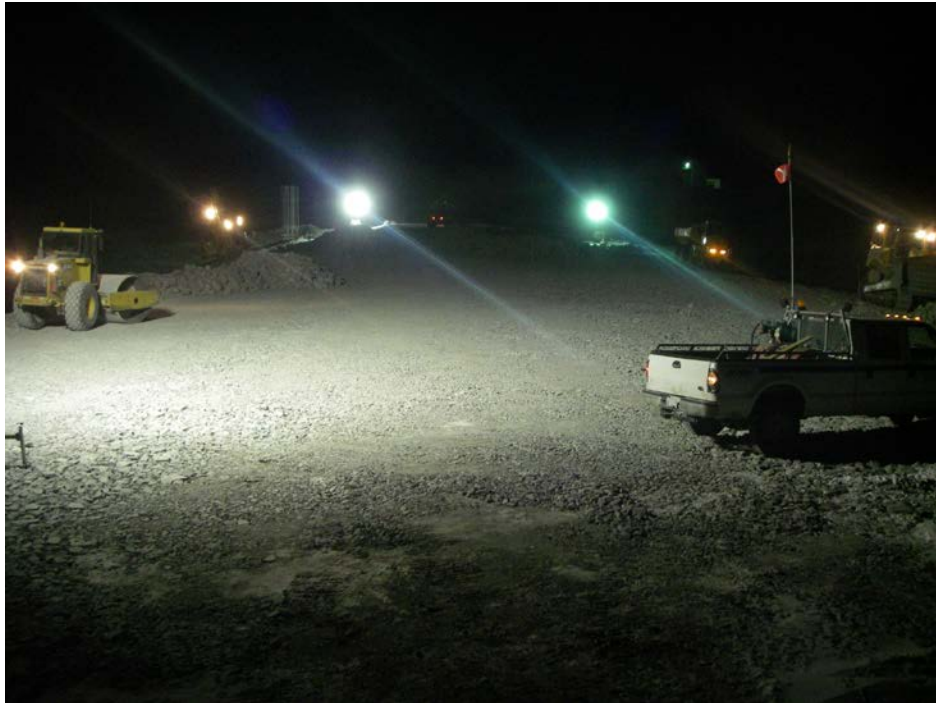
Photo 11: North Dam – completed third lift of ROQ. Compactor is compacting the ROQ as well as the transition surfaces. Photo taken from Sta.0+10, looking north-east.
