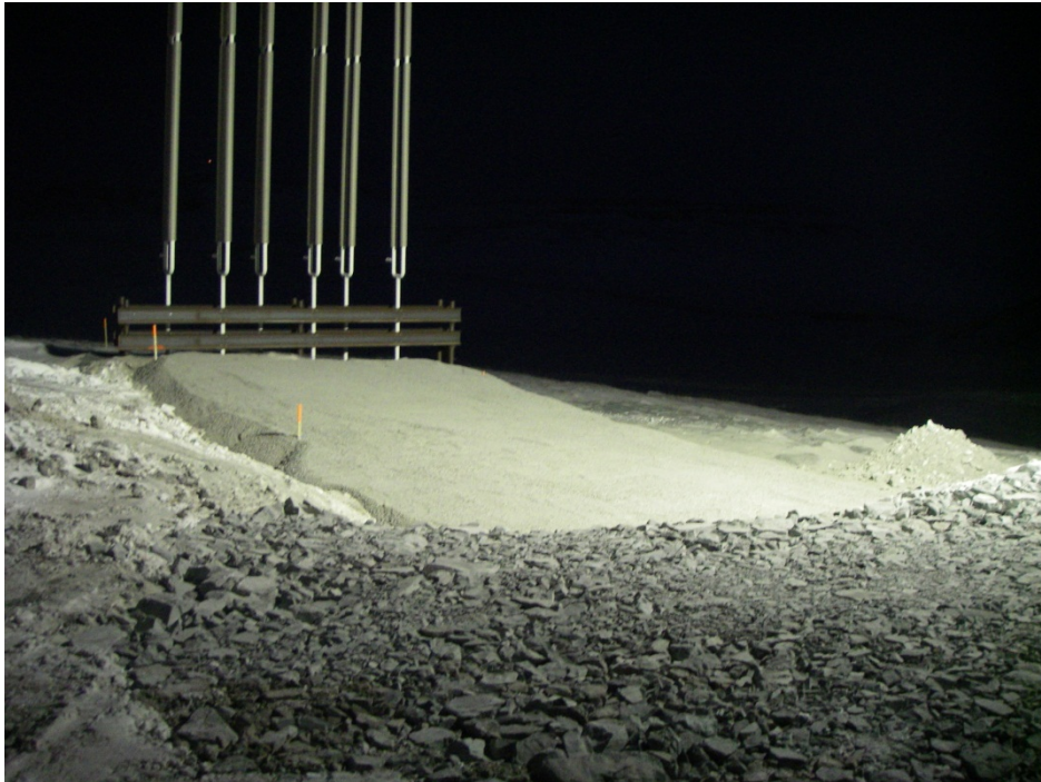
Photo 9: North Dam – completed crush placement at the south thermosyphon radiators. Photo looking west.
