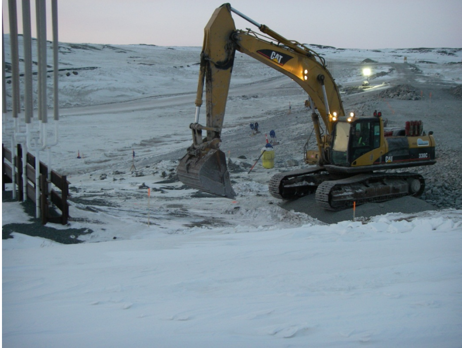
Photo 8: North Dam – excavator clearing snow before additional crush placement at south thermosyphon radiators. Photo looking north-east.
