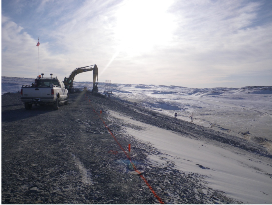
Photo 4: North Dam – View of progress on north dam. Line and stakes mark the final crest which is at grade.
