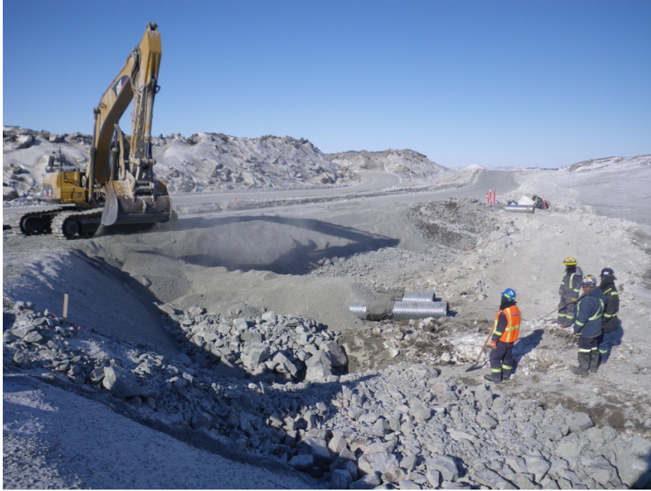
Photo 6: Diversion Berm – Culverts after placement of first lift of ROQ and crush material.
