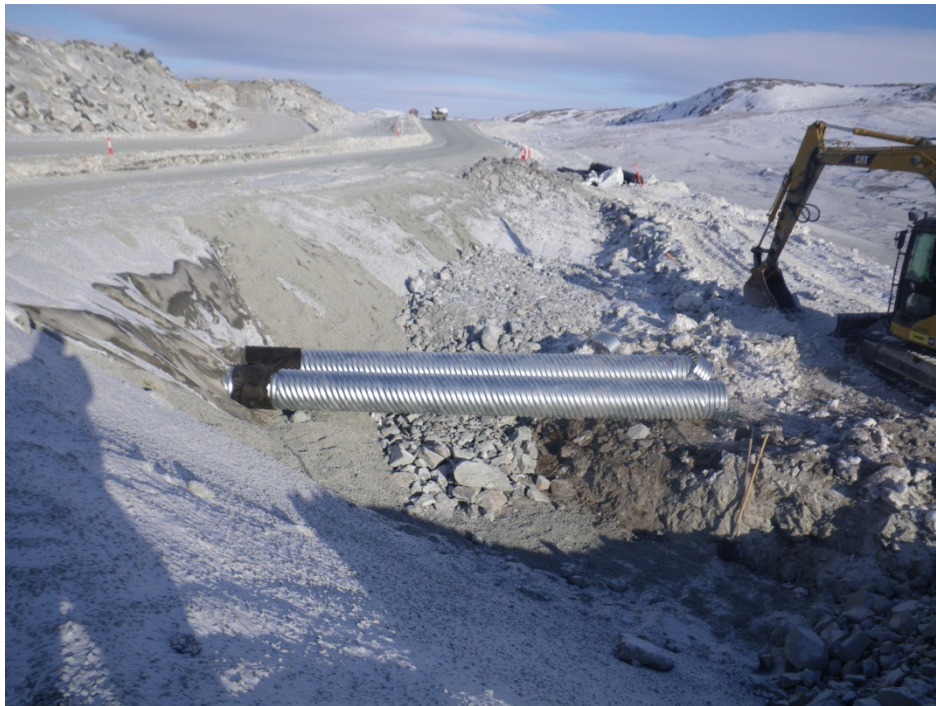
Photo 5: Diversion Berm – Culvert extensions installed at crossing through Primary Road.
